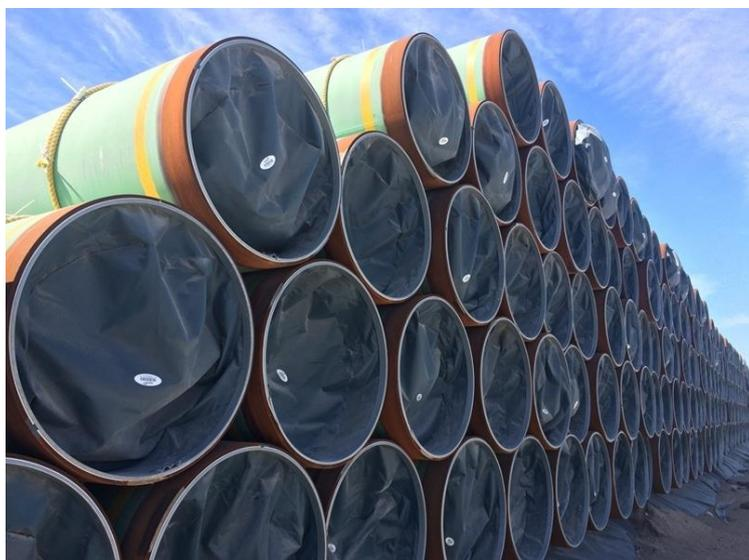
*“Within our environment you can never guarantee that tags do not get damaged or lost. Luckily our pipes have two end caps so that we can fit tags to both sides. As a back-up we also have the unique identification of the pipe itself. Creating redundancy is extremely crucial in our environment.”*
