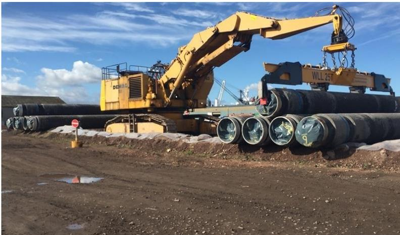
*ShawCor has fitted the 'spreader bar' of heavy lift machines with an all-in-one box with RFID-reader, DGPS-modem (Differential Global Positioning System) and 4G/WIFI modem - which enables the machine to read and trace the tags every time a pipe is included.*
